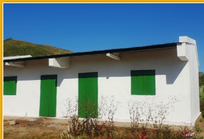
Rehabilitation of the Ambohipo school © HELPSIMUS
