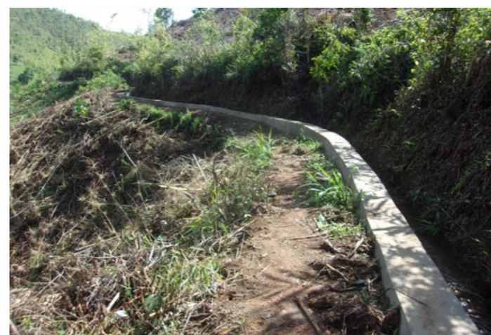
Irrigation improvement works © IMPACT Madagascar
