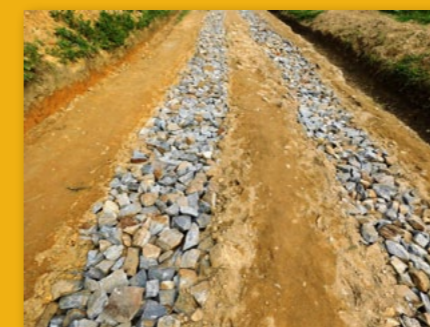
Repair of the main track © HELPSIMUS
