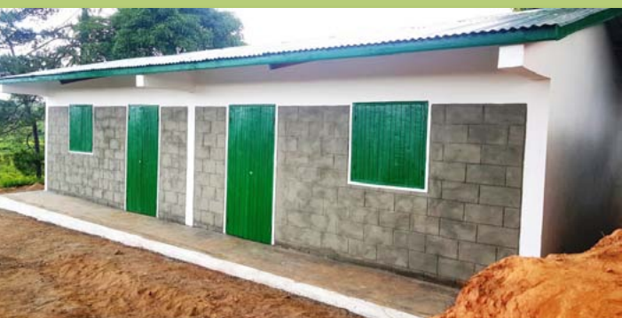
New building at the school of Vohitrarivo © HELPSIMUS
