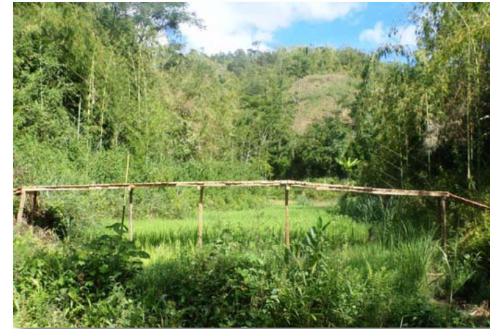
Footbridge on the territory of Group 2 © HELPSIMUS
