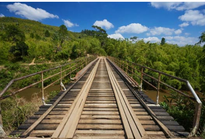
Large Bridge after Renovation © S. Meys
