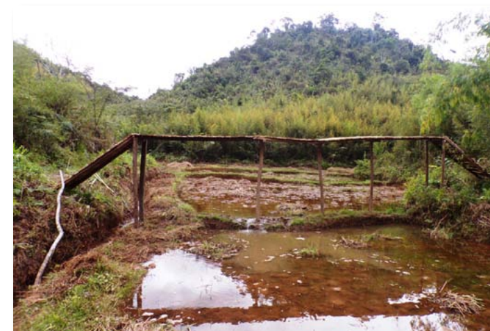
Footbridge on the territory of Group 1 © HELPSIMUS
